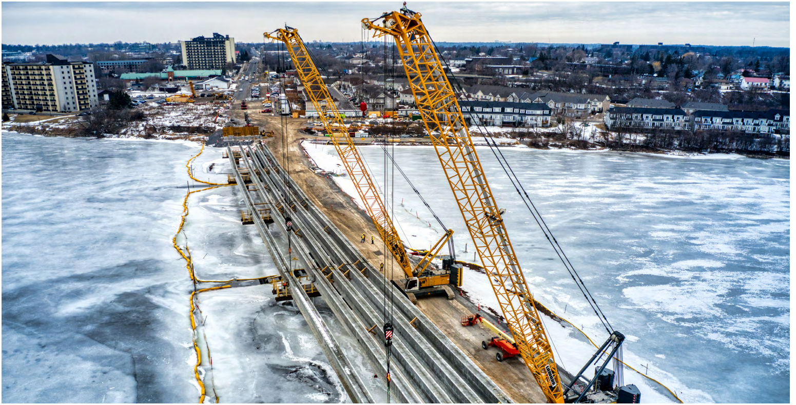
Two Cranes Sitting On The Temporary Causeway
