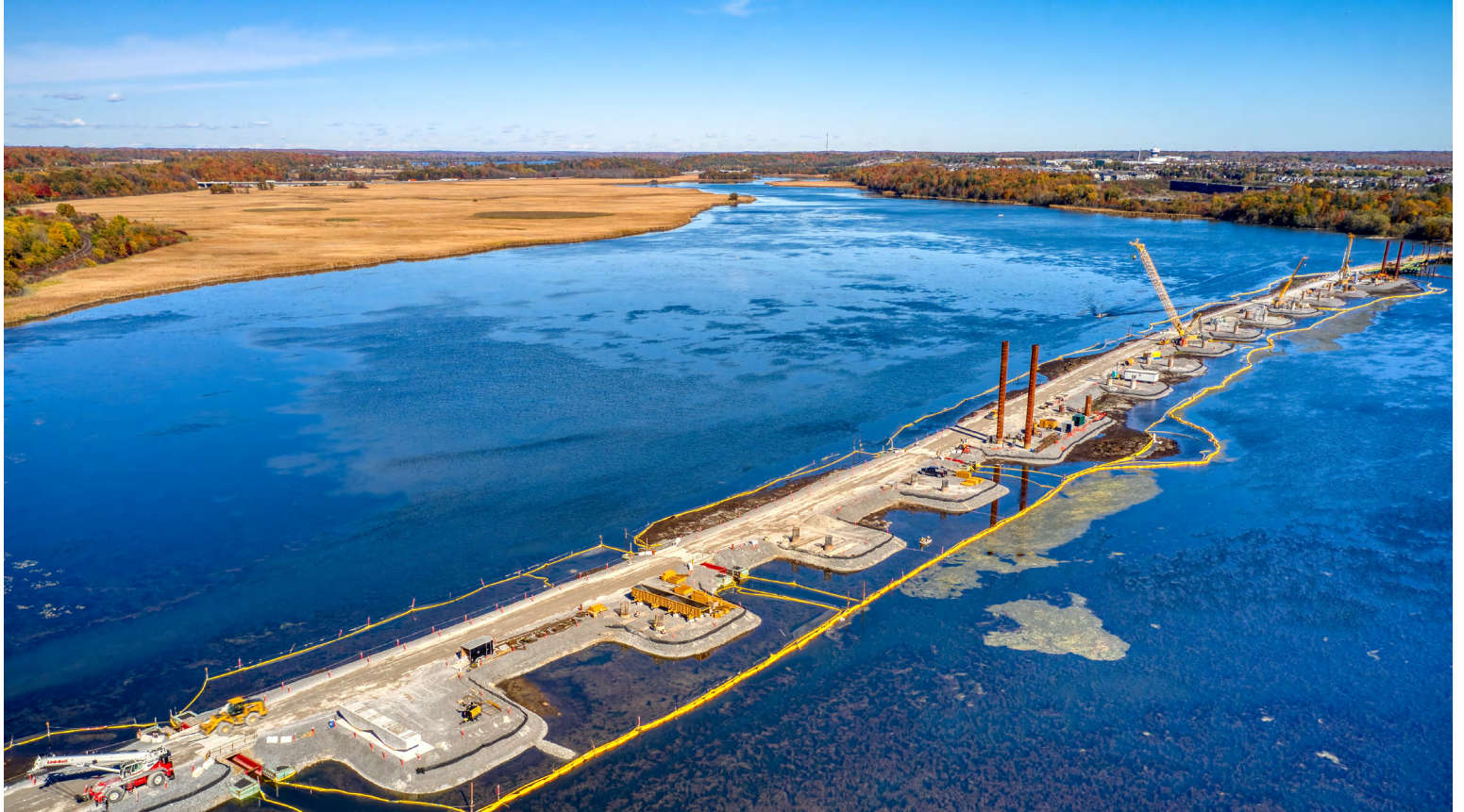
Piles And Pile Caps Being Constructed
