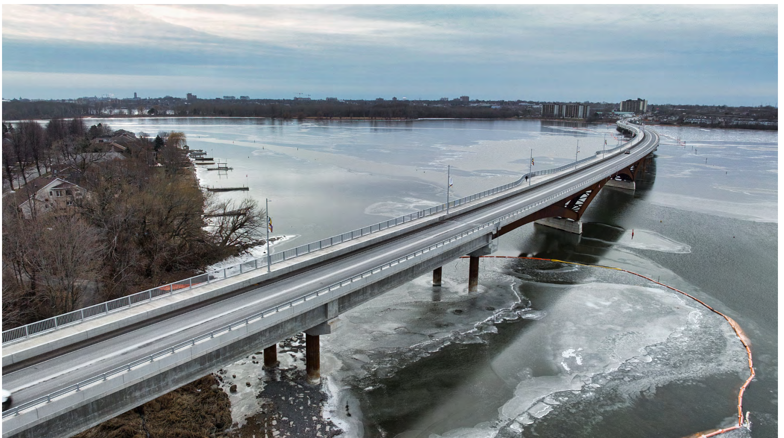
The Waaban Crossing, Opened To Traffic
