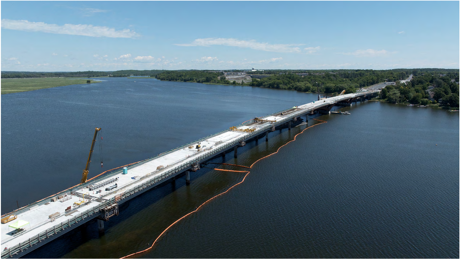
An Overview Of The Eastern End Of The Bridge
