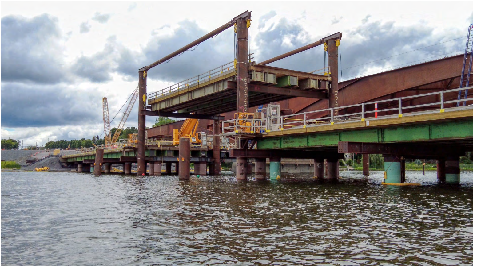
The Temporary Lift-Bridge Over The Cataraqui
