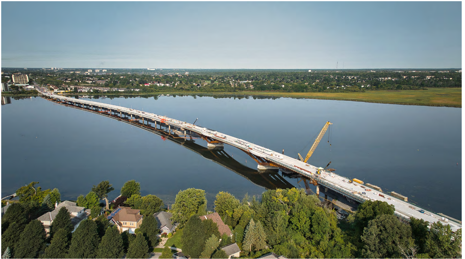
The Bridge Looking Westwards
